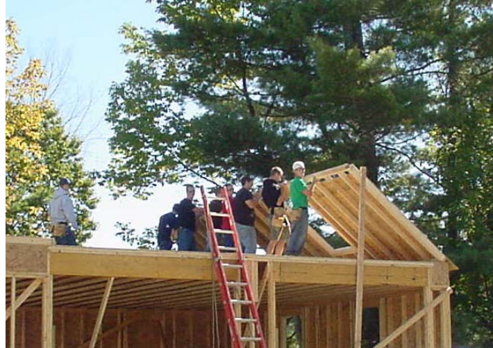
Below: Raising the walls on the second floor
